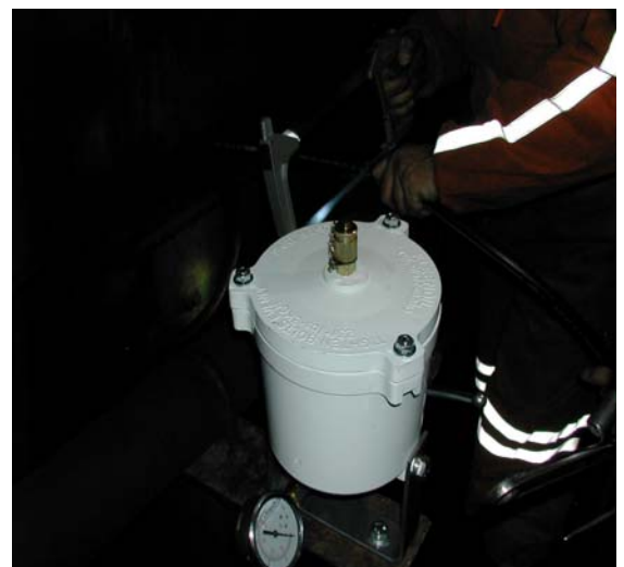
9778UMZ on Dodge Rockwell CST. Installed 7km underground on coal transfer conveyor
